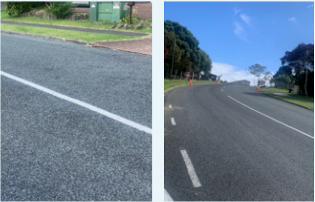
Examples of chip sealing in Unsworth Heights, North Shore, three weeks after the seal went down
