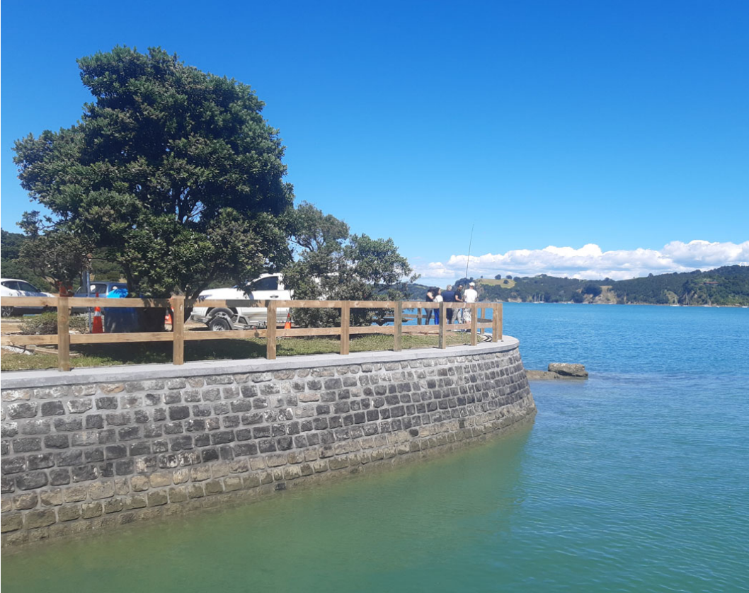
Figure 9: Scotts Landing Seawall Renewal
