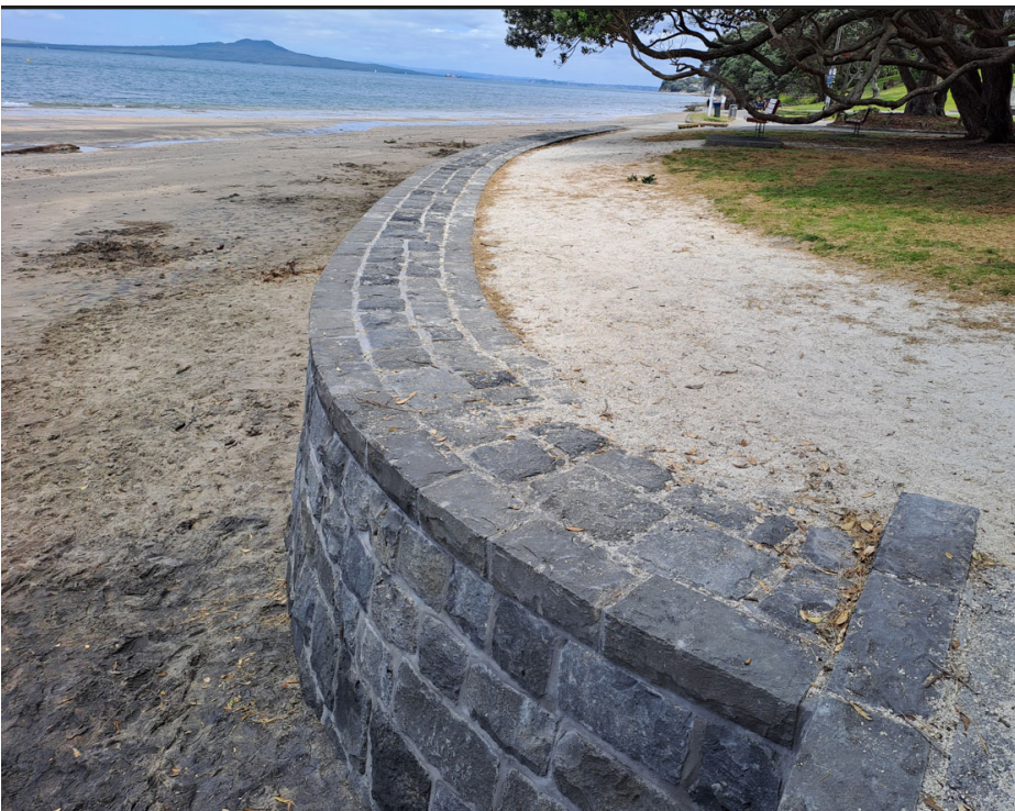
Figure 4: New masonry rock seawall completed in September 2023
